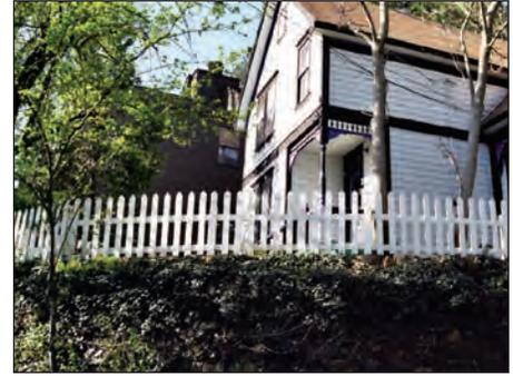
*Picket fence over high stone retaining wall*
