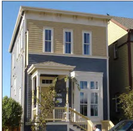
*Contemporized form with bay window, portico, spindle railing and cornice details*
