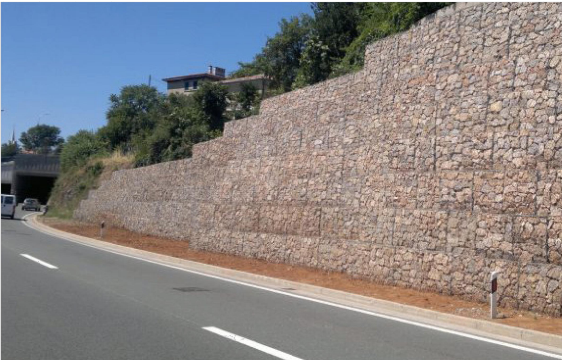
GABION WALLS ALONG HIGHWAYS
