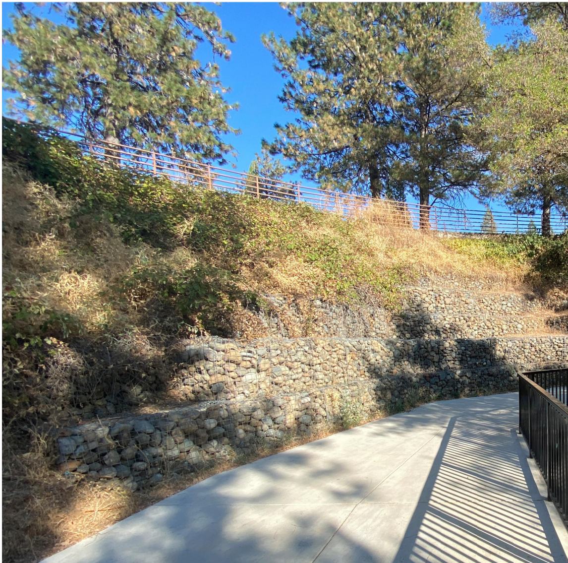
EXISTING GABION WALLS AT NORTHSTAR MINING MUSEUM
