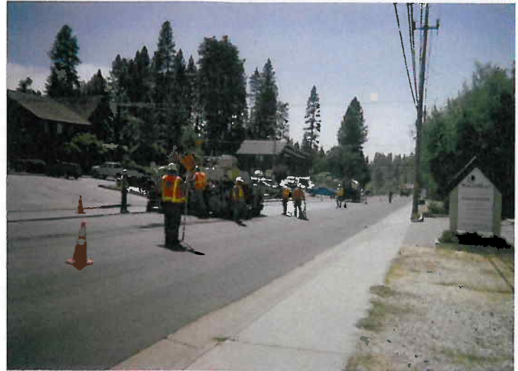
- VIEW - East Main Street (looking south towards Presley Way)
