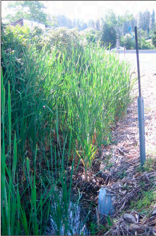
4a. Vegetated roadside ditch.
