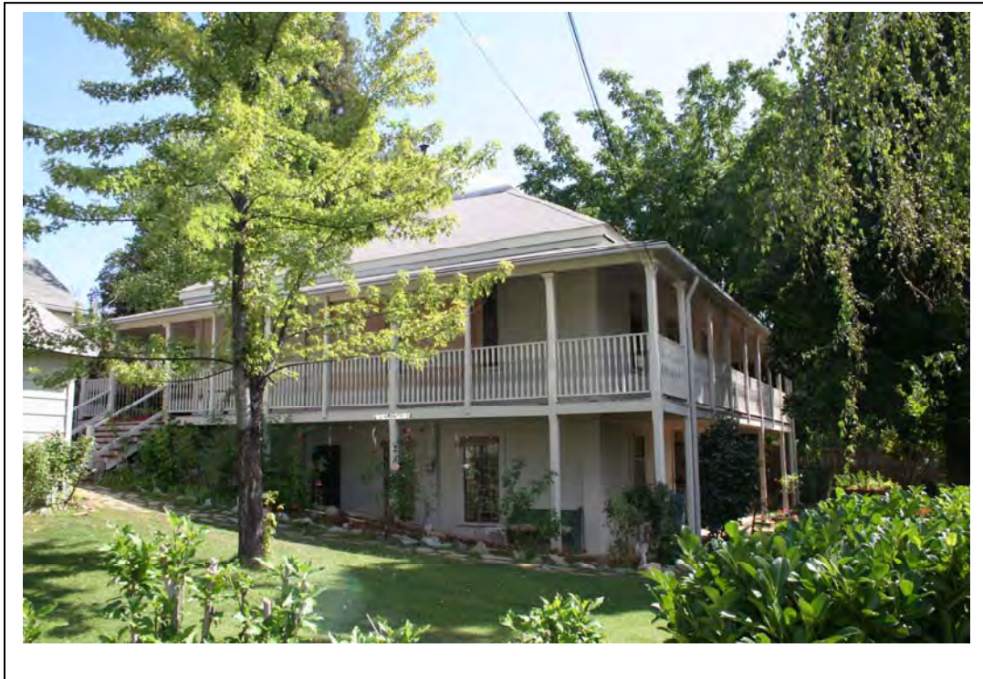
Rare vernacular rammed earth residence at the intersection of Bennett and Kidder streets.
