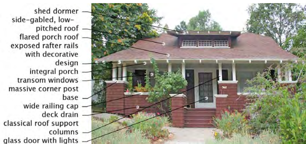
Architectural detail of a Craftsman residence
