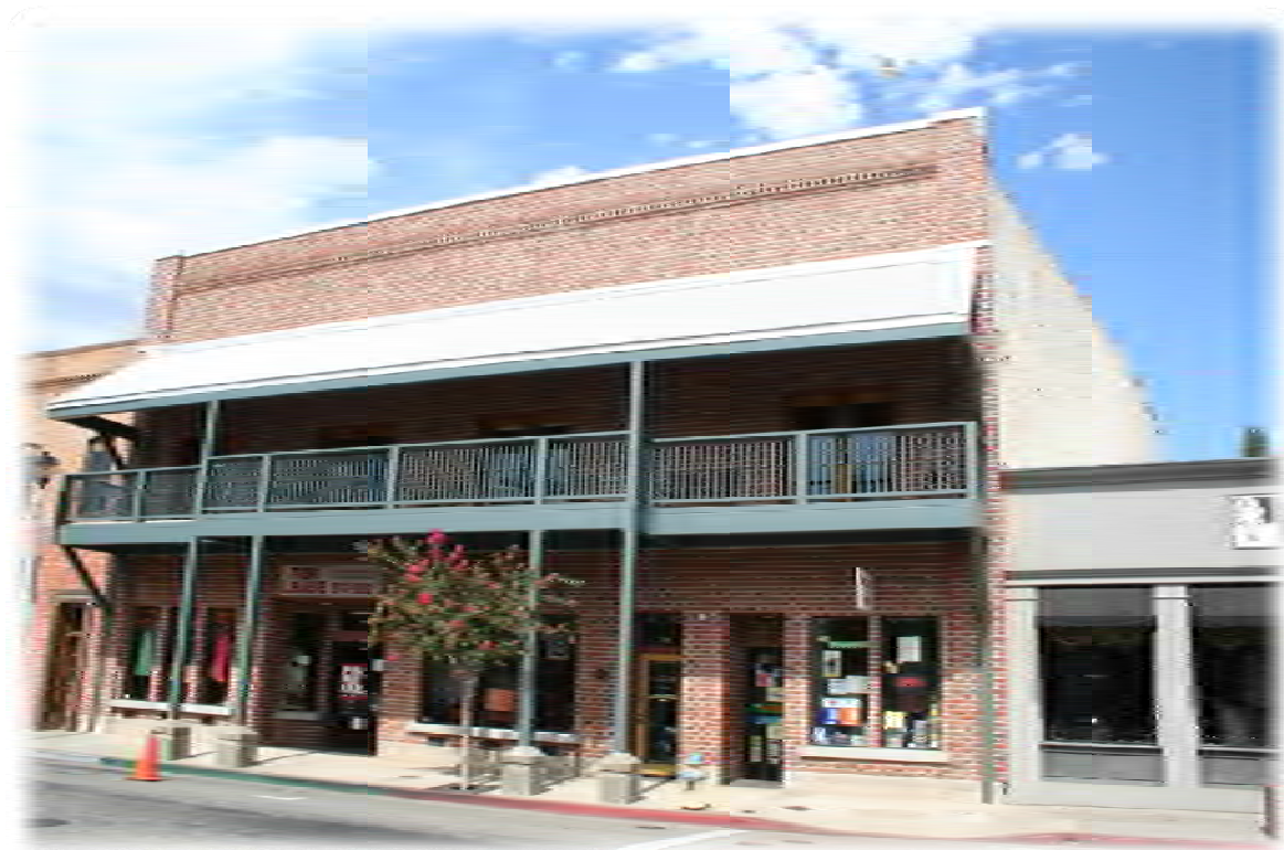
Rehabilitated commercial storefront facing E. Main Street.
