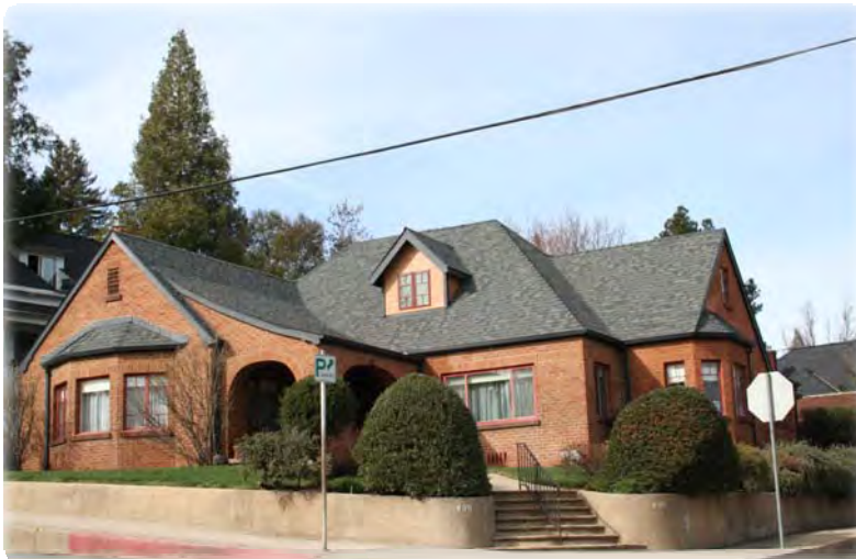
An example of English Cottage Revival design along W. Main Street exhibiting many important design elements emphasizing the use of brick, arches, bays, steep gables, and hipped roofs to create an attractive residence. This home, built in 1926 for Ernest and Clara George, was restored after a recent fire.
