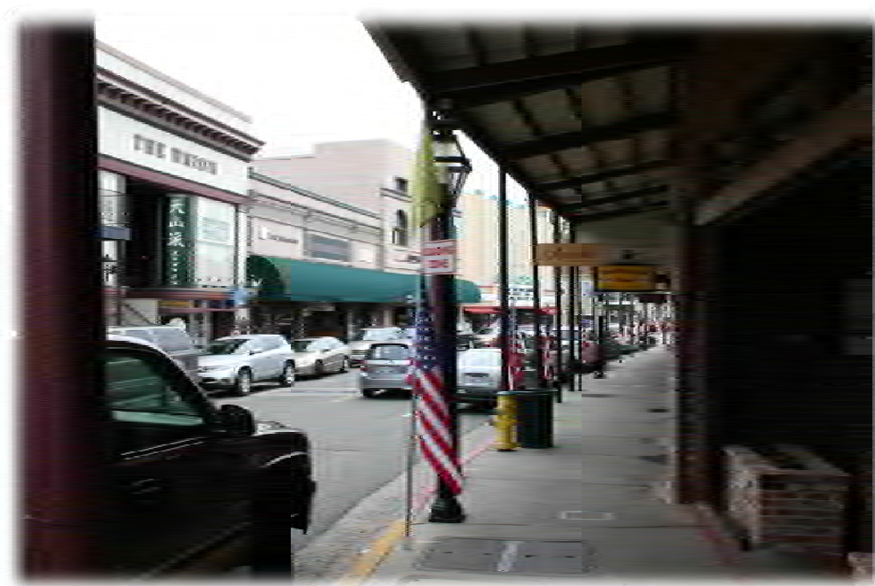
Row of circa 1890s wood and metal roof, and steel column verandas along the west side of Mill Street.
