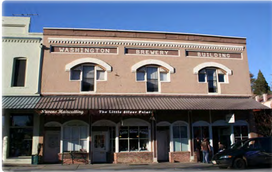
Note the flat parapet, use of arched lintels to dress the windows, and row of brick dentils below the belt course on the Washington Brewery Building facing E. Main Street.
