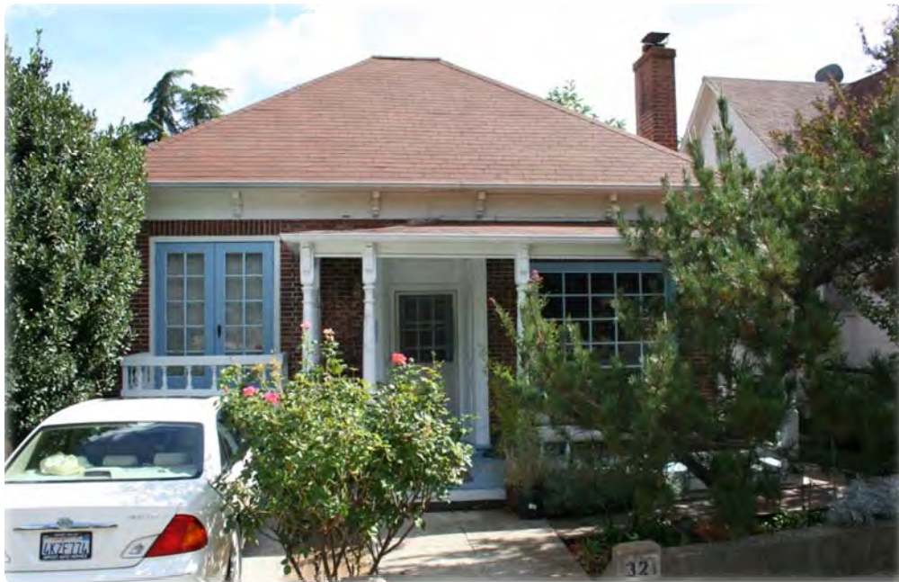
Rare mid-Victorian (circa 1870) brick hipped roof residence. Note the more recent window alterations.
