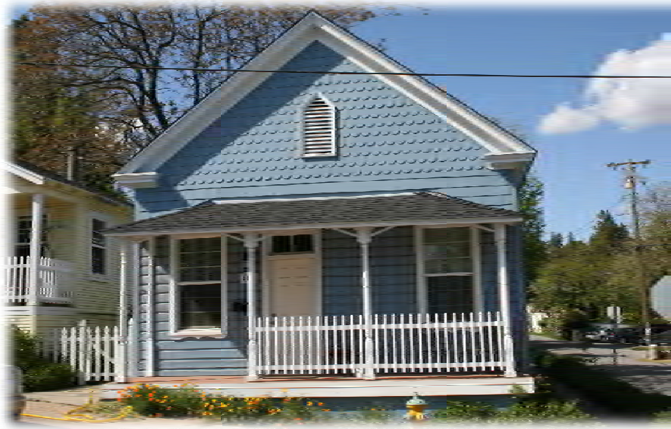
Replacement porch on a circa 1860s Late Victorian residence
