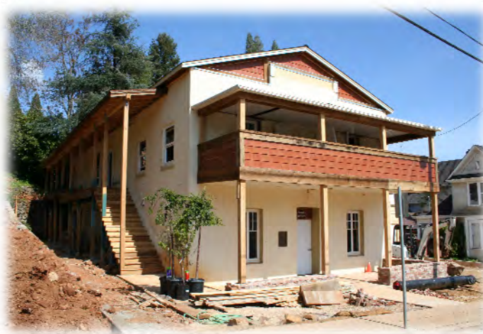
Rehabilitation involving reuse of historic fabric and replacement materials that match the building's original design and fabric.
