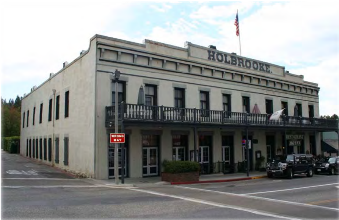
A handsome Classical Revival brick masonry hotel known as the Holbrooke on West Main Street. Note the stepped parapet roof and repetition in the cornice windows and doors.
