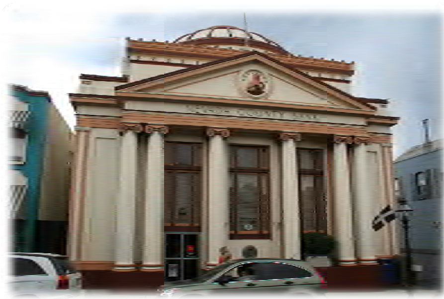
The elegant Neo-Classical Nevada Bank Building.
