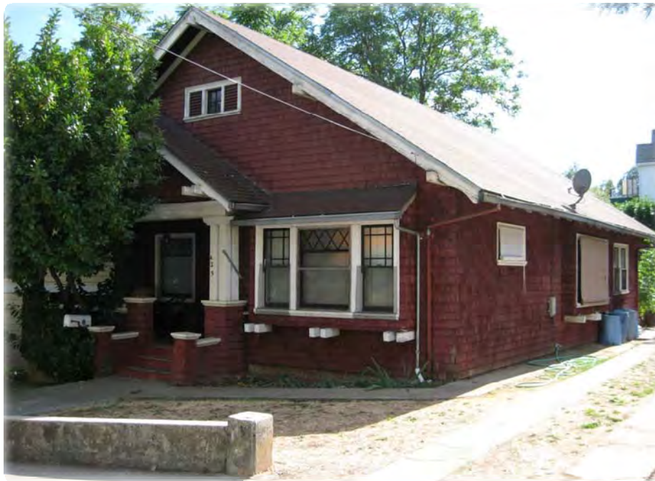
Another front gable Craftsman with shingle exterior cladding. The triple window with divided sashes typifies this house type.
