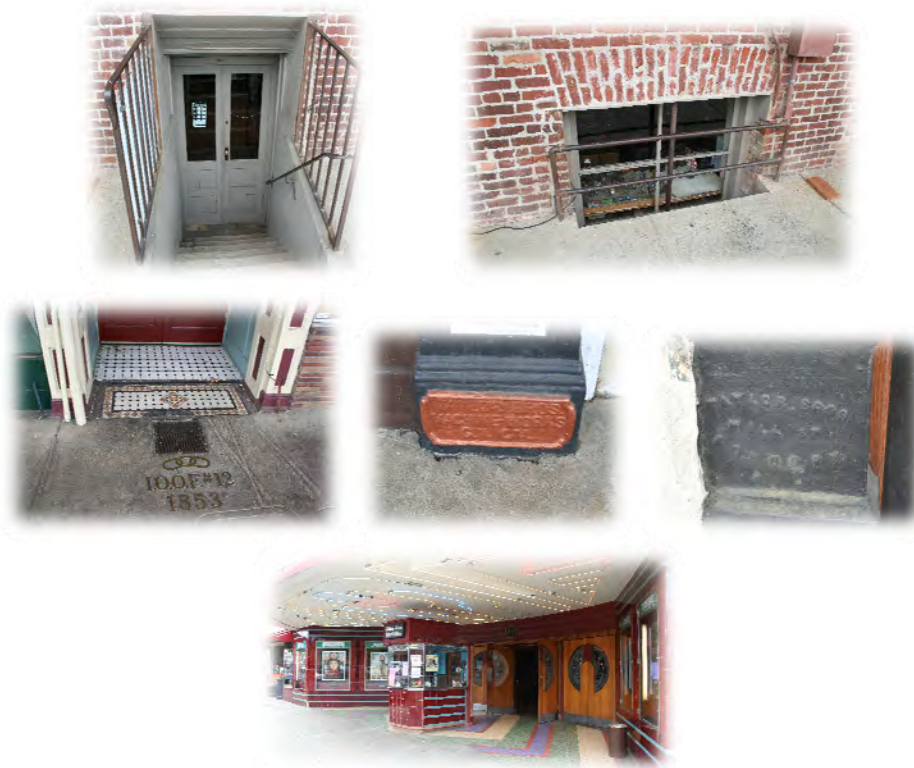
Architectural detail of Grass Valley commercial storefronts: (Top left) Below grade entrance; (Top right) Below grade window detail (Middle left) Ornate tile entry IOOF Hall; (Middle center) Iron pilaster manufactured by Taylor Bros. Machine Works, Grass Valley (Middle right) Cast iron frieze made by Taylor Bros at the base of a pilaster; and (Bottom center) Restored Art Deco Del Oro theater entrance and ticket booth.
