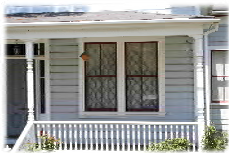
Original paired wood-sash windows with 2 over 2 lights
