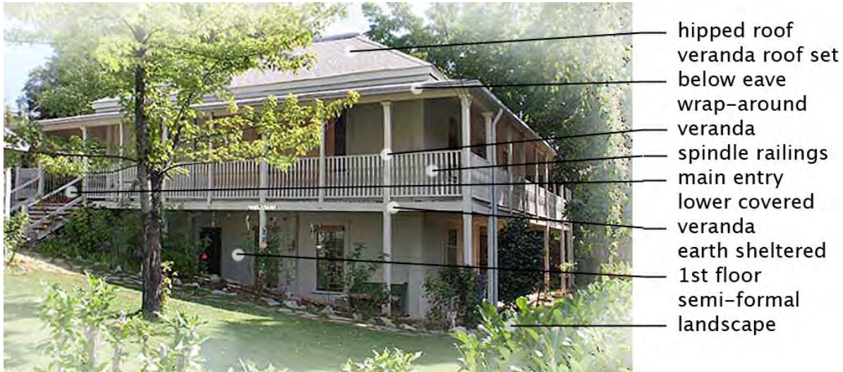
Typical details of a Late Victorian Residence
