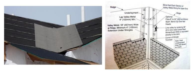
Open valleys are those in which the roof-covering material stops several inches short of the centerline of the valley. The valley is protected from moisture intrusion by a W valley flashing. Minimum 24" wide 26 gauge, metal installed over galvanized/coated 72 # Cap Sheet or 90 # roll roofing.
